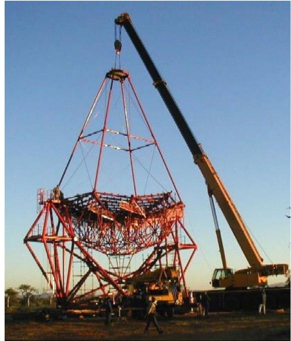
**Fig. 2.** The last step in the assembly of the structure of the first telescope is the mounting of the camera support.
