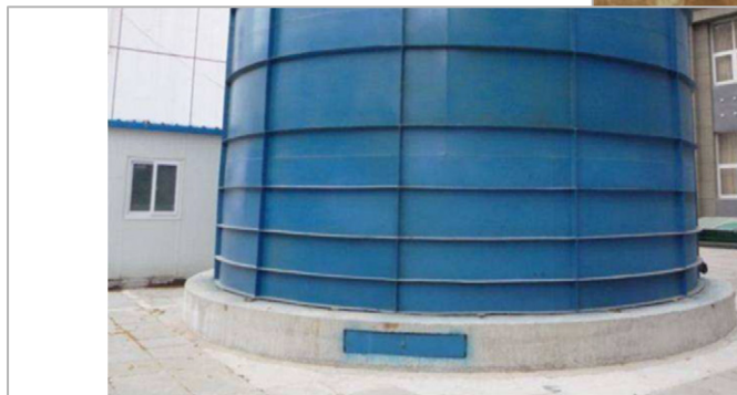
Fig. 1. Picture of the prototype water Cherenkov detector. It is a cylinder tank, 7.07 m in diameter and 5.00 m in height.
