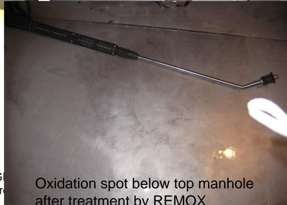
Oxidation spot below top manhole after treatment by REMOX
