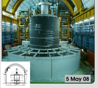
**(below right)** All vertical surfaces within the water tank including those of the cryostat have been covered with a reflective and wave-length shifting foil for improved detection of the Cherenkov light. The purple layer on the cryostat's wall consists of 6mm thick extruded poly-styrene foam serving as a thermal impedance which limits the evaporation in case of a leak in the inner container. A similar barrier is mounted on the inner wall.
