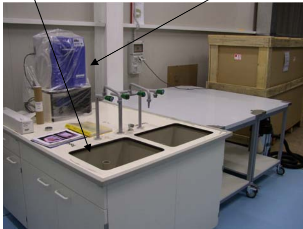
Washstand with high-purity water supply
