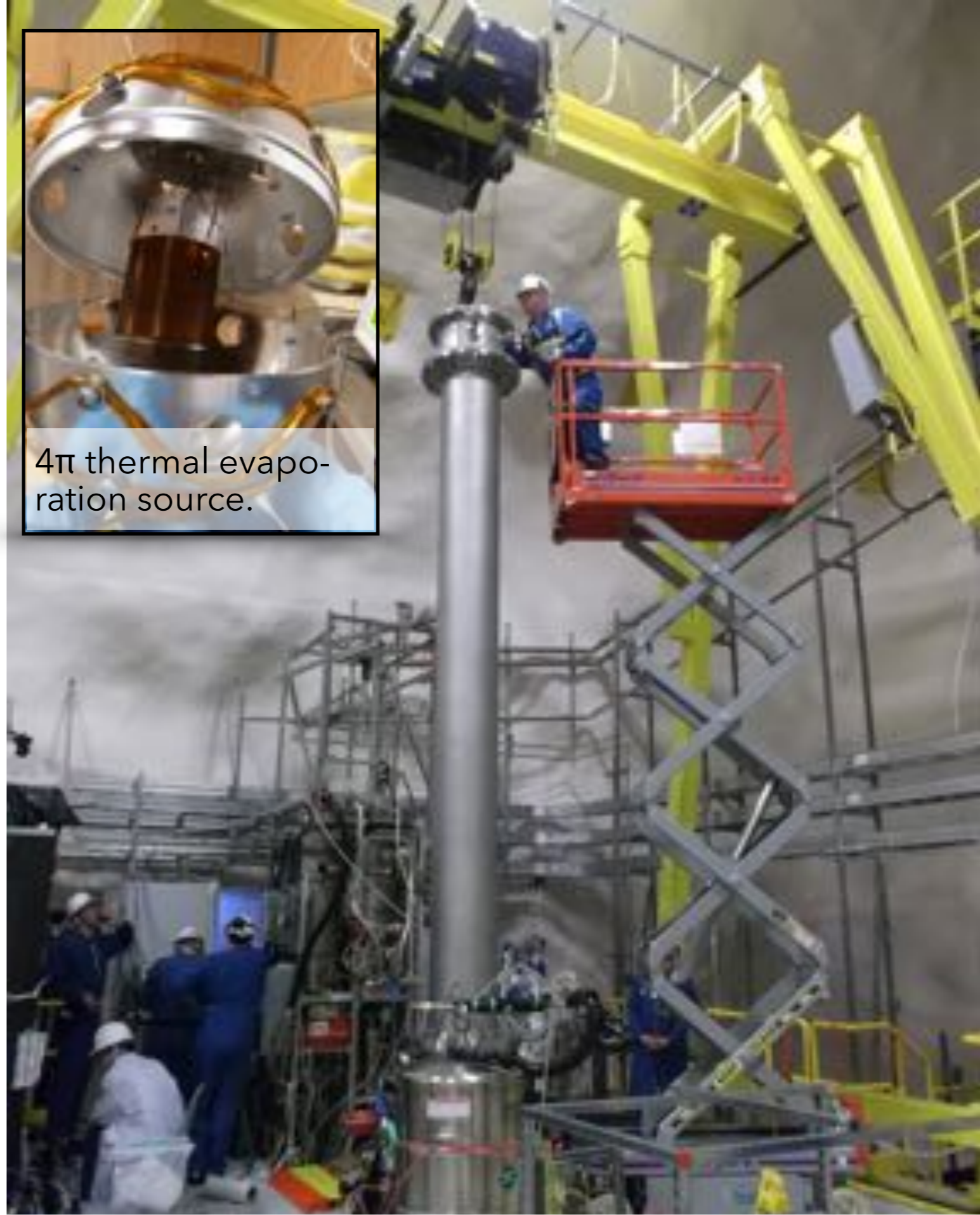
TPB deposition system being installed.
