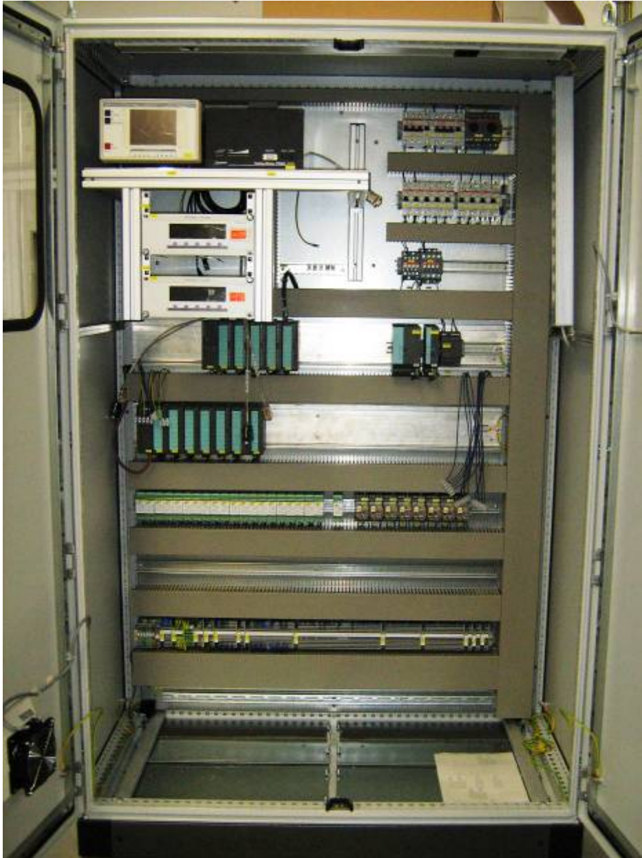
PLC at MPI Heidelberg
