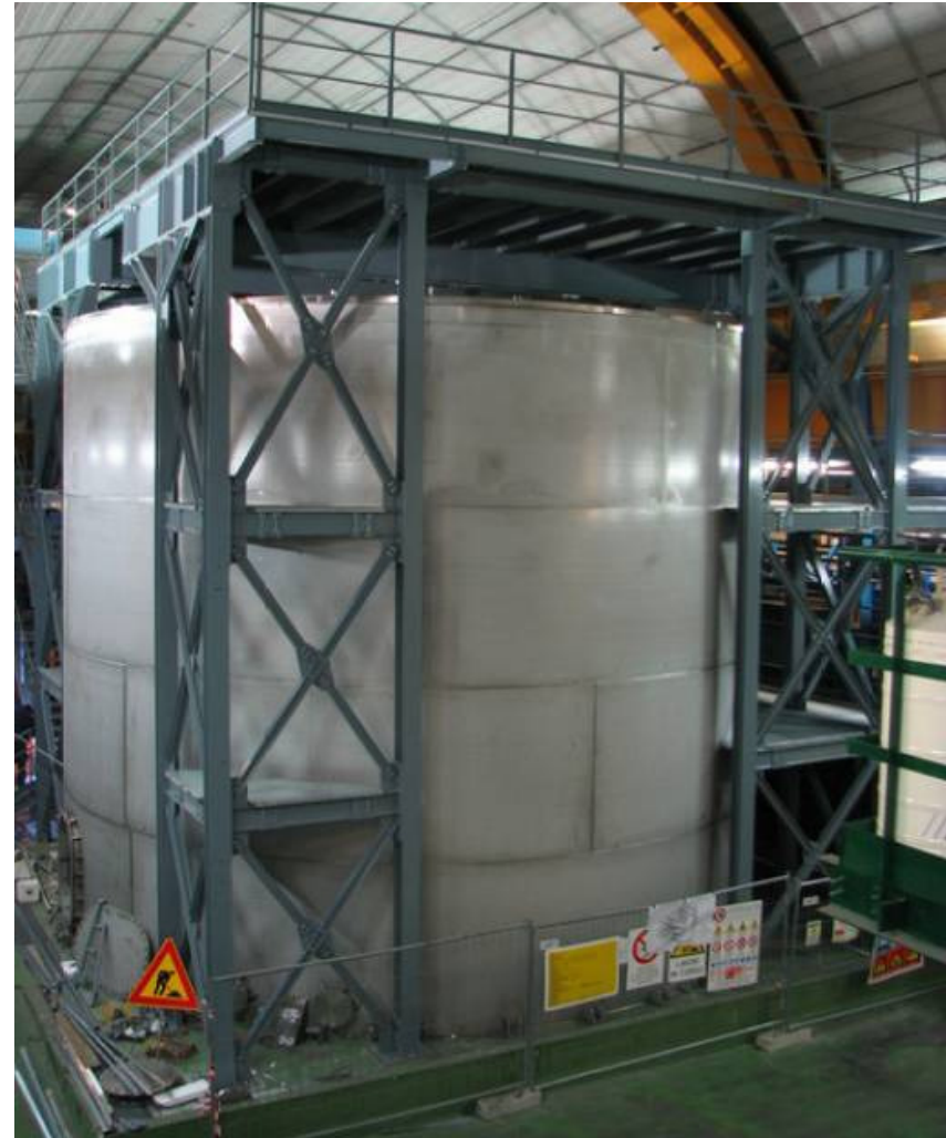
water tank (Aug. 2008)
