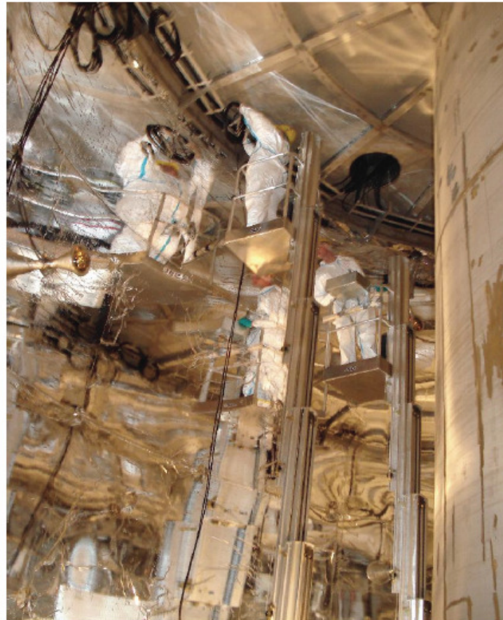
PMT installation inside Water Tank (May 2009)
