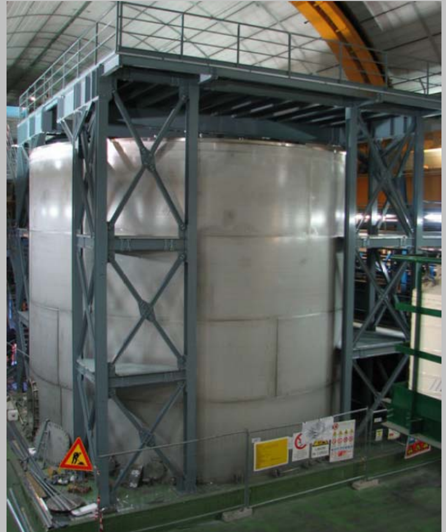
water tank (Aug.2008)
