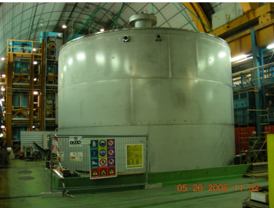
Water tank installation: April - June 2008
