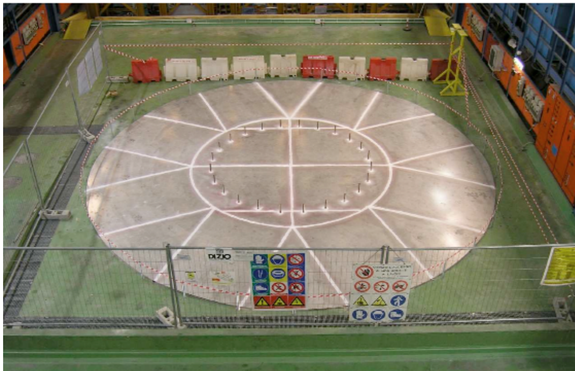
August 2007, floor plate for water tank
