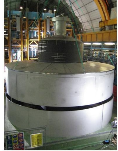
Figure 4. The construction of the GERDA water tank on May 2008
