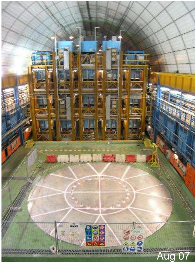
Ready for cryostat installation on bottom plate of water tank (hall A in front of LVD).
