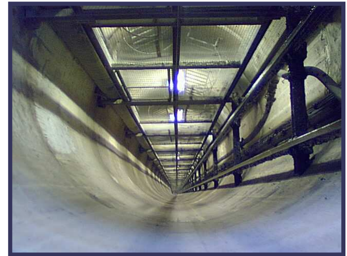
During the refurbishment process, the diodes are stored underground, in Hades facility, Geel, Belgium
