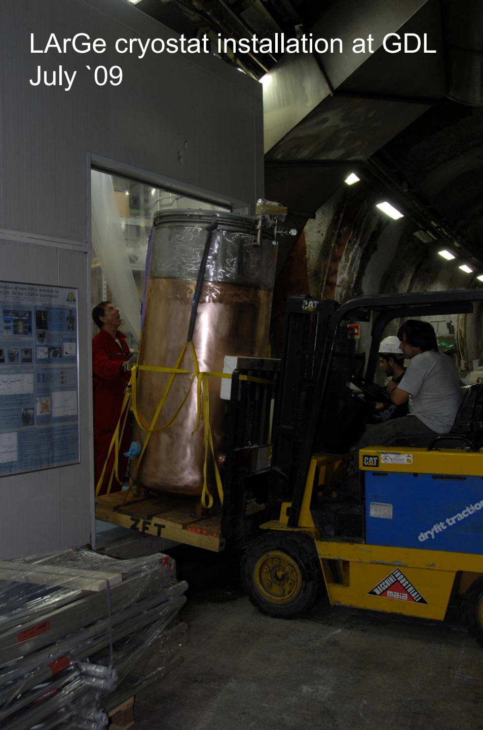
insertion of the cryostat into the shielding
