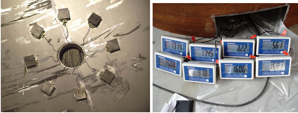
Figure 8: The 8 load cells arranged on the support pads at the bottom of the outer vessel (left), and the measured loads (in kg) on the individual pads after the inner vessel has been lowered onto the pads. The stiffness of the Belleville spring below each pad is 59 kN / mm.
