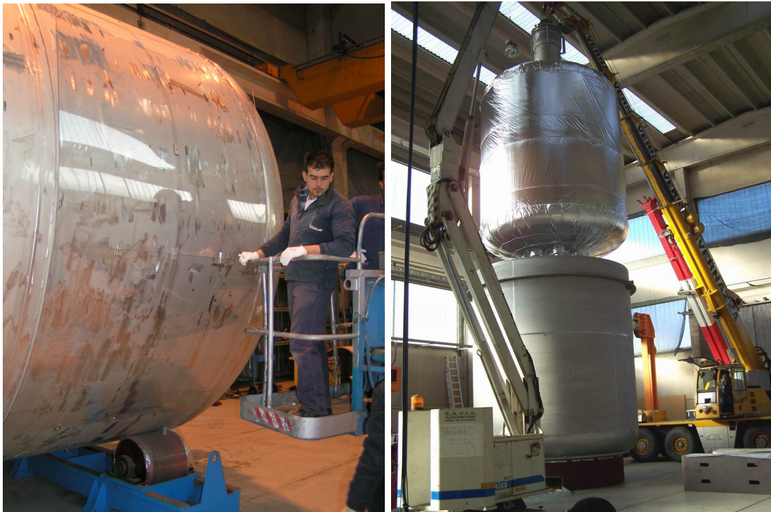
Figure 7: Mounting of the Makrolon sheets onto the outer surface of the inner vessel (left), and insertion of the inner vessel (covered by the multilayer insulation) into the outer vessel.
