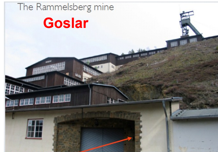
Entry to the shaft
